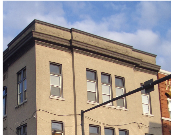
25. Flat roof concealed behind parapet (Source: ERA Architects)
