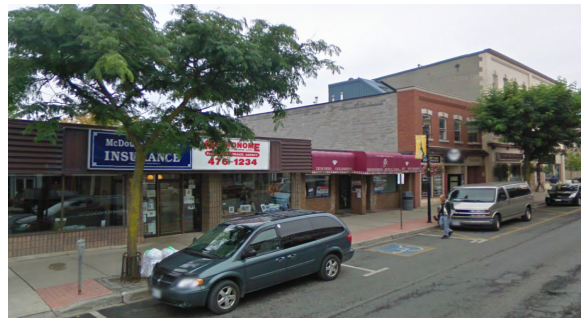
22. 1-storey post-war retail buildings disrupt the consistent street wall and diminish the sense of enclosure. (Source: Google Streetview)
