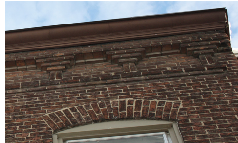
36. Original entablature at 204 Main Street (Source: ERA Architects)
