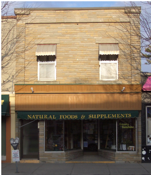
38. Concealing modern equipment, such as solar panels, behind parapets may be an appropriate method of conserving the heritage attributes of the District (Source: ERA Architects)
