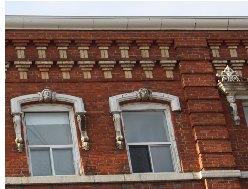
35. Cast iron window hoods on 237 Main Street (Source: ERA Architects)
