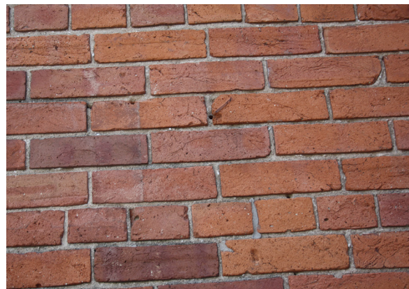
34. Brick is a high quality and durable material that is commonly found in the District (Source: ERA Architects)
