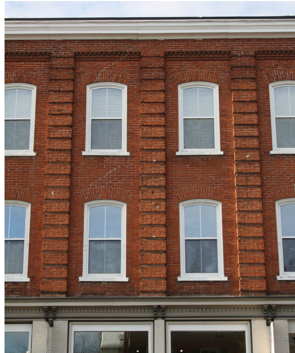
23. Rusticated pilasters divide the front façade into bays at 171/173 Main Street (Source: ERA Architects)
