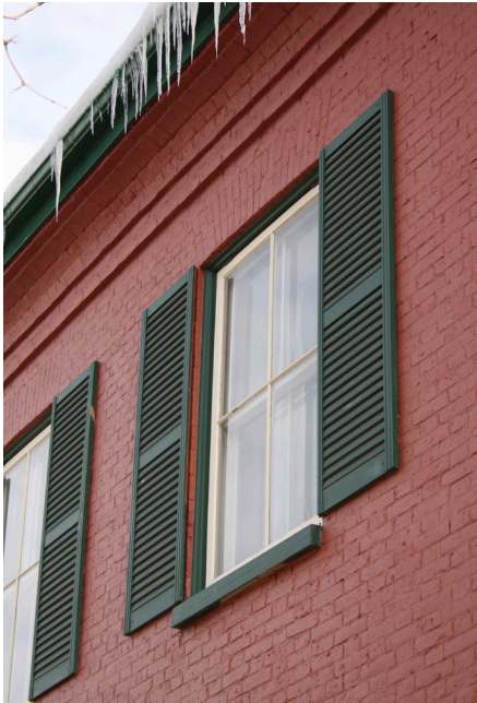
27. Example of compatible secondary glazing at 172 Main Street (Source: ERA Architects)
