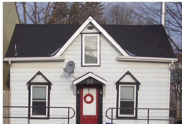
26. Pitched roof on residential building (Source: ERA Architects)
