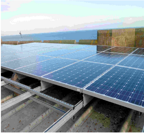
37. Solar panels concealed behind a parapet at Lindisfarne Castle, England (Source: National Trust, ntenvironmentalwork.net)
