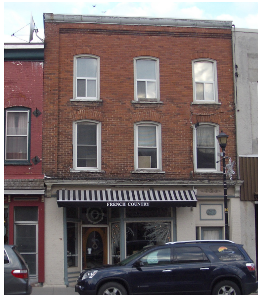
32. Retractable awning does not obscure architectural detail, such as the storefront cornice at 255/257 Main Street (Source: ERA Architects)
